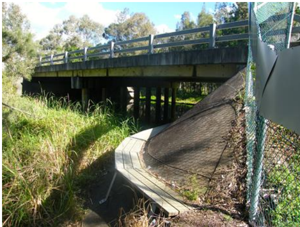
FIGURE 3 EXAMPLE OF KOALA/FAUNA WALKWAY ADDITION TO ROAD BRIDGE UNDERPASS (SOURCE: D. JONES 2013)
