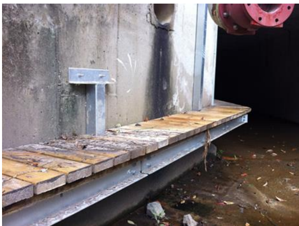
FIGURE 2 EXAMPLE OF KOALA/FAUNA WALKWAY ADDITION TO CULVERT (SOURCE: D. JONES 2013)
